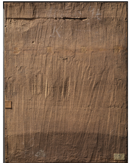
Fig. 3 Reverse with original coating in raking light.
